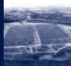
3 MWp PV plant near Teruel
