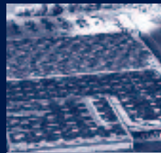
Industrial roof system
